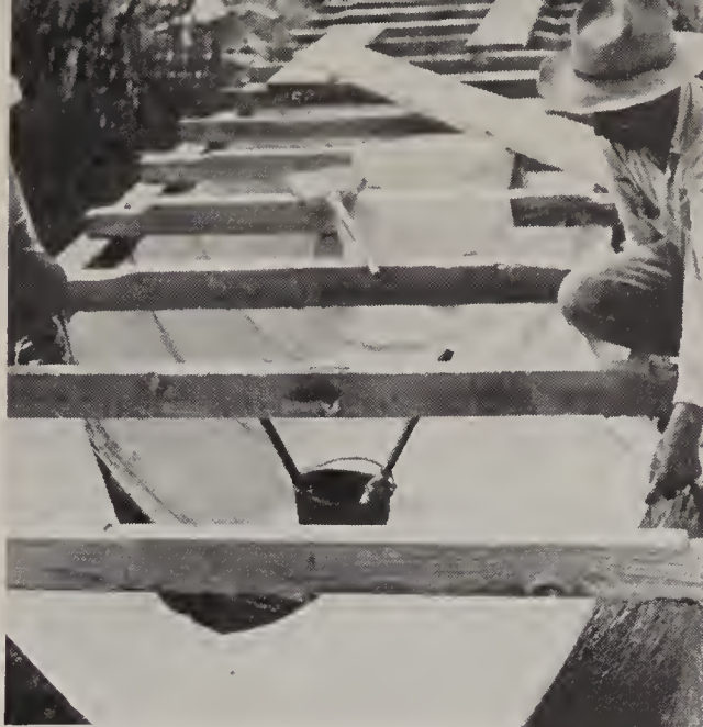
Special-warp cotton fabric is applied with asphalt for repairing metal flume.
